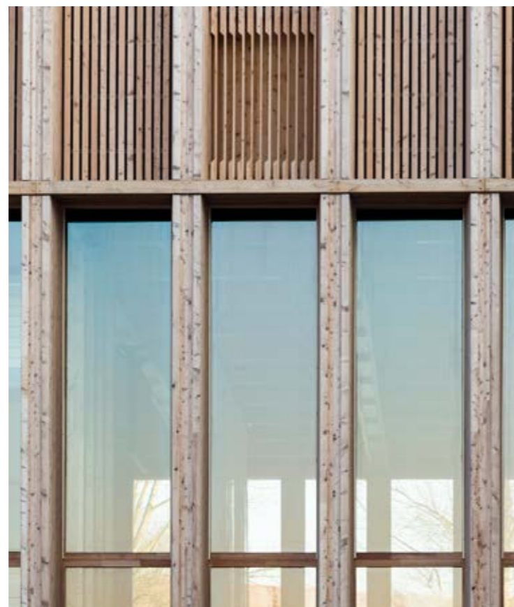
A2 "Gymnase" is a sports hall in Strasbourg
